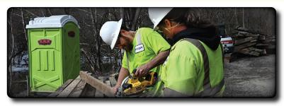
Workers are replacing each board on the wooden deck one at a time. It takes eight boards placed side by side to make up a foot of bridge deck, so the entire 420-foot bridge will require about 3,360 individual boards.
