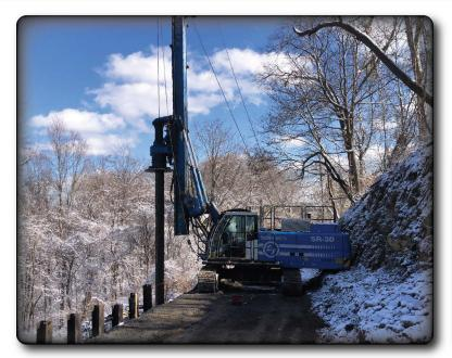
West Virginia Division of Highway (WVDOH) crews were hard at work in District 3, Pleasants County. Crews were installing steel piling wall beams to help provide lateral support for the roadway slope, this support helps to prevent future road slips. Thanks for all your hard work and for keeping our roadways safe for the traveling public!
