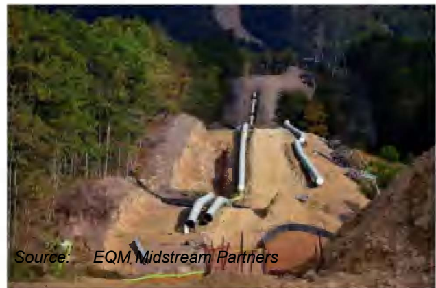
Figure 2-10 Pipeline Under Construction in West Virginia
