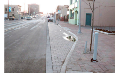
Parking Delineation with Concrete Band
