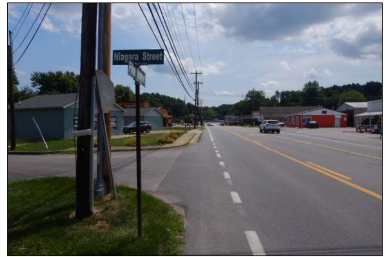
Photo 50: Facing south along the east side of WV 14 at Niagara Street.
