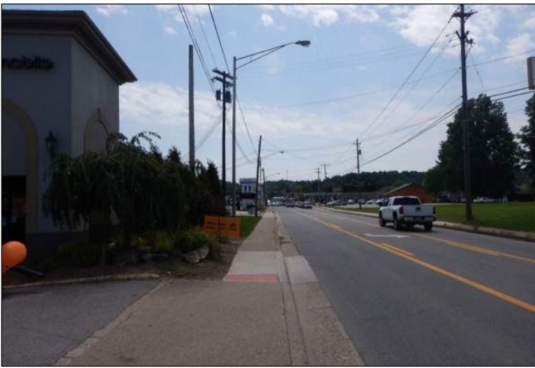
Photo 17: Facing south along the east side of WV 14.
