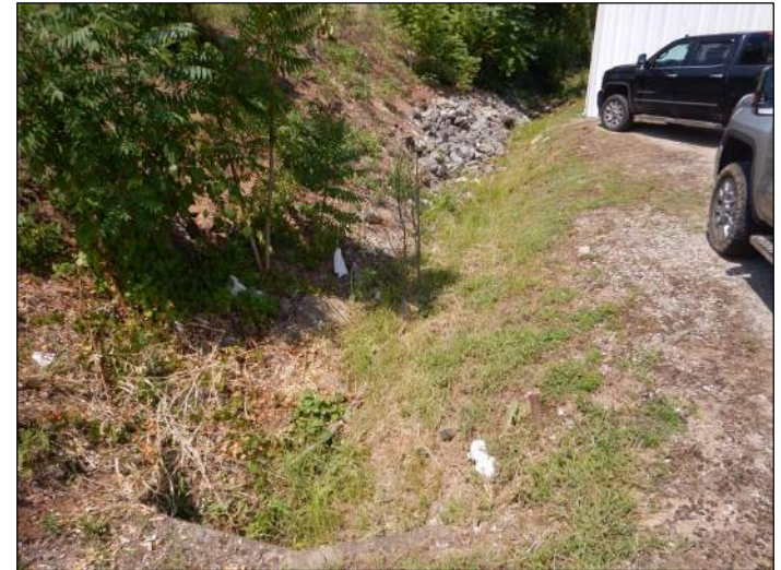
Photo 4: Facing north along a riprap ditch that feeds into the culvert inlet/outlet.
