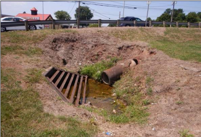
Photo 3: Between Blizzard Drive and WV 14 at a culvert outlet/inlet.
