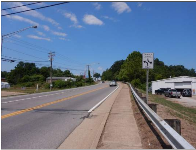
Photo 5: Facing northwest along Blizzard Drive at the northern end of the project..
