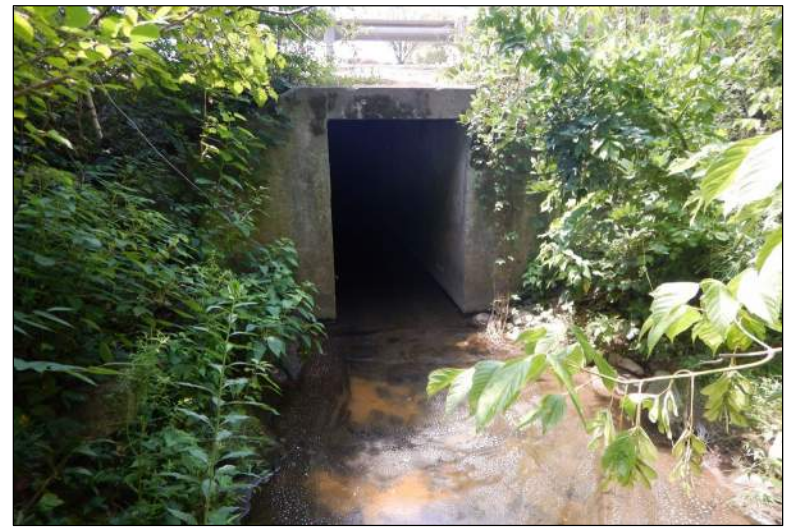
Photo 46: Facing west at the outlet of UNT to Wards Run.
