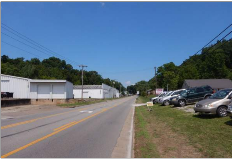
Photo 1: Facing north along WV 14 at the northern end of the project.
