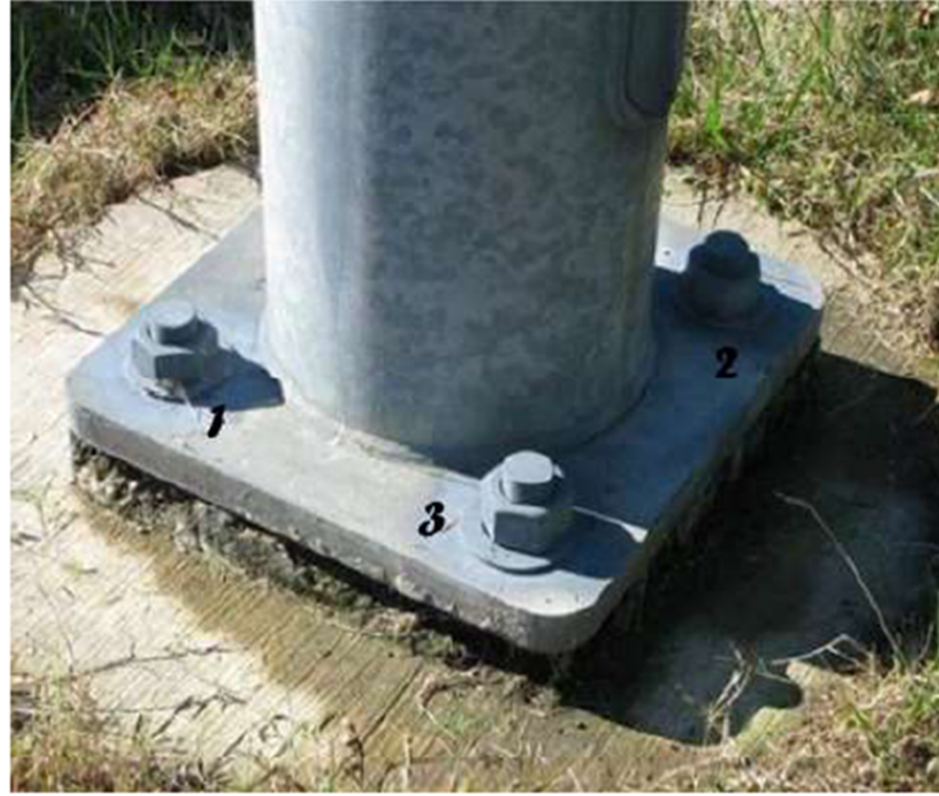
FIGURE 2 -SNUG TIGHTENING SEQUENCE NUMBERING ON BASE PLATE
