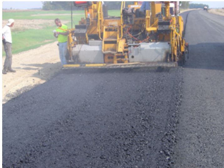
Figure 39 – Truck Segregation Effects
