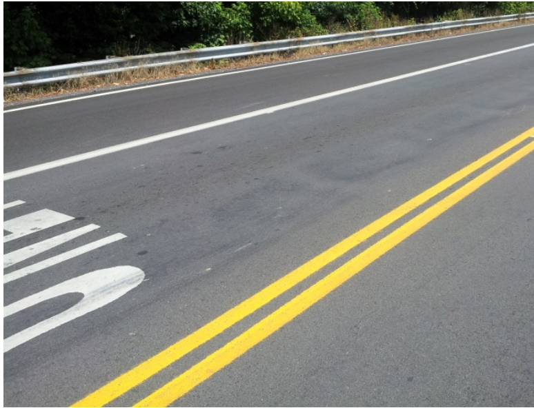
Excessive rutting and shoving in new asphalt pavement. Note the displacement of the road lettering. Also note the presence of corresponding flushing of liquid asphalt.
