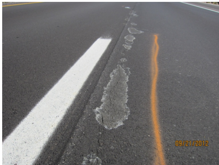
Tear in new asphalt pavement. Note water stains along cracks. Area has been marked for repair.
