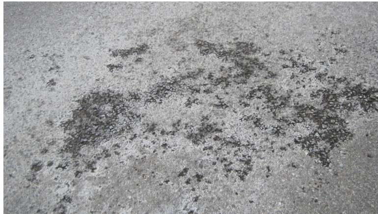
Photo shows advanced raveling and segregation of a Superpave 12.5 mm mix.
