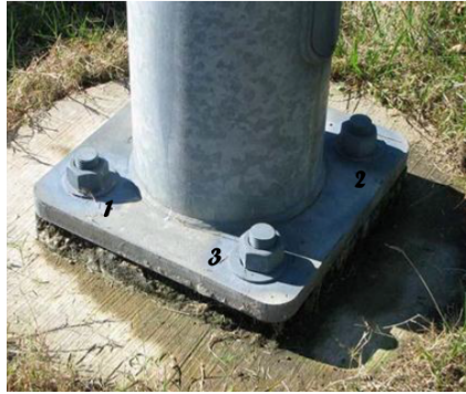
SNUG TIGHTENING SEQUENCE NUMBERING ON BASE PLATE
