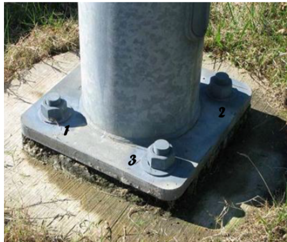
SNUG TIGHTENING SEQUENCE NUMBERING ON BASE PLATE
