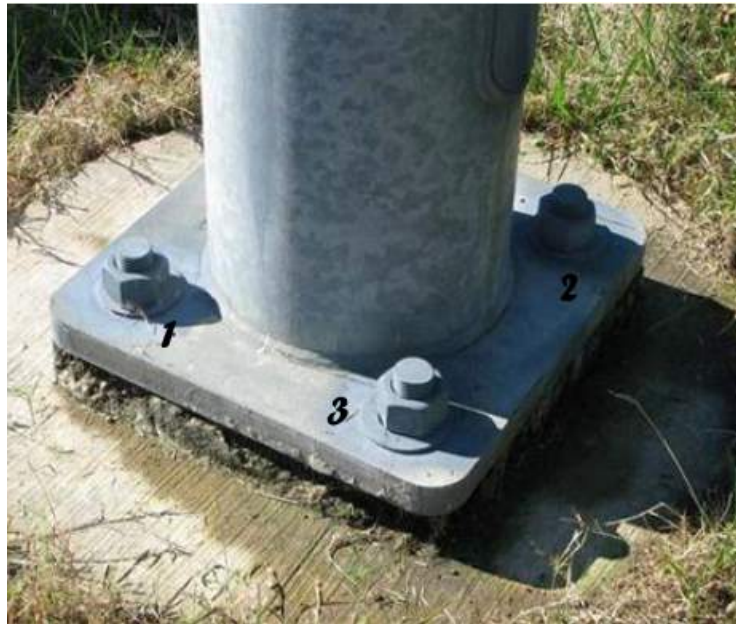
FIGURE 2 -SNUG TIGHTENING SEQUENCE NUMBERING ON BASE PLATE
