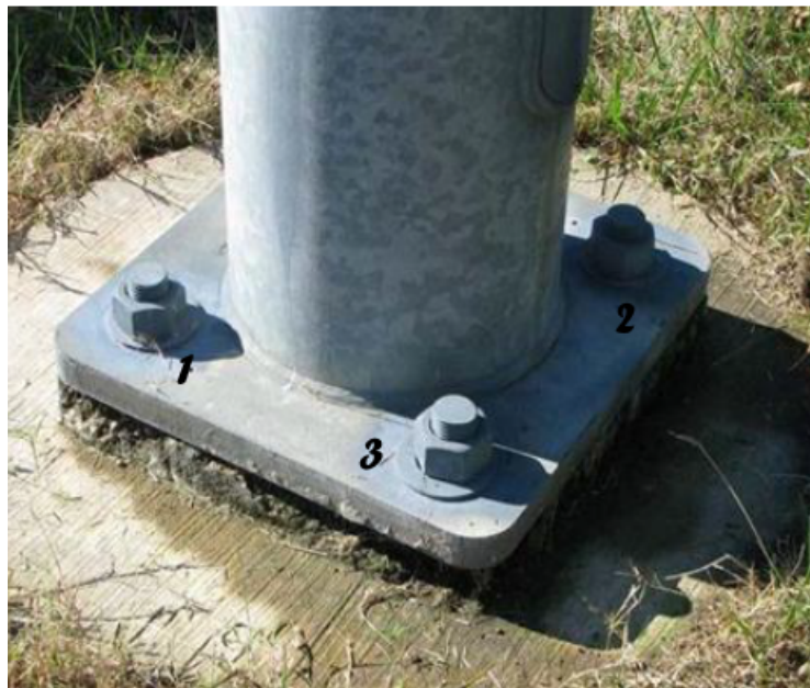
Figure 2 -Snug Tightening Sequence Numbering On Base Plate
